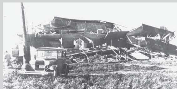
Figure 2. Photograph of a wood-frame building in Long Beach, California destroyed by the March 11, 1933 earthquake. Photo credit: Seismicity of the United States, 1568-1989 (Revised) , by Carl W. Stover and Jerry L. Coffman, U.S. Geological Survey Professional Paper 1527, United States Government Printing Office, Washington: 1993.
